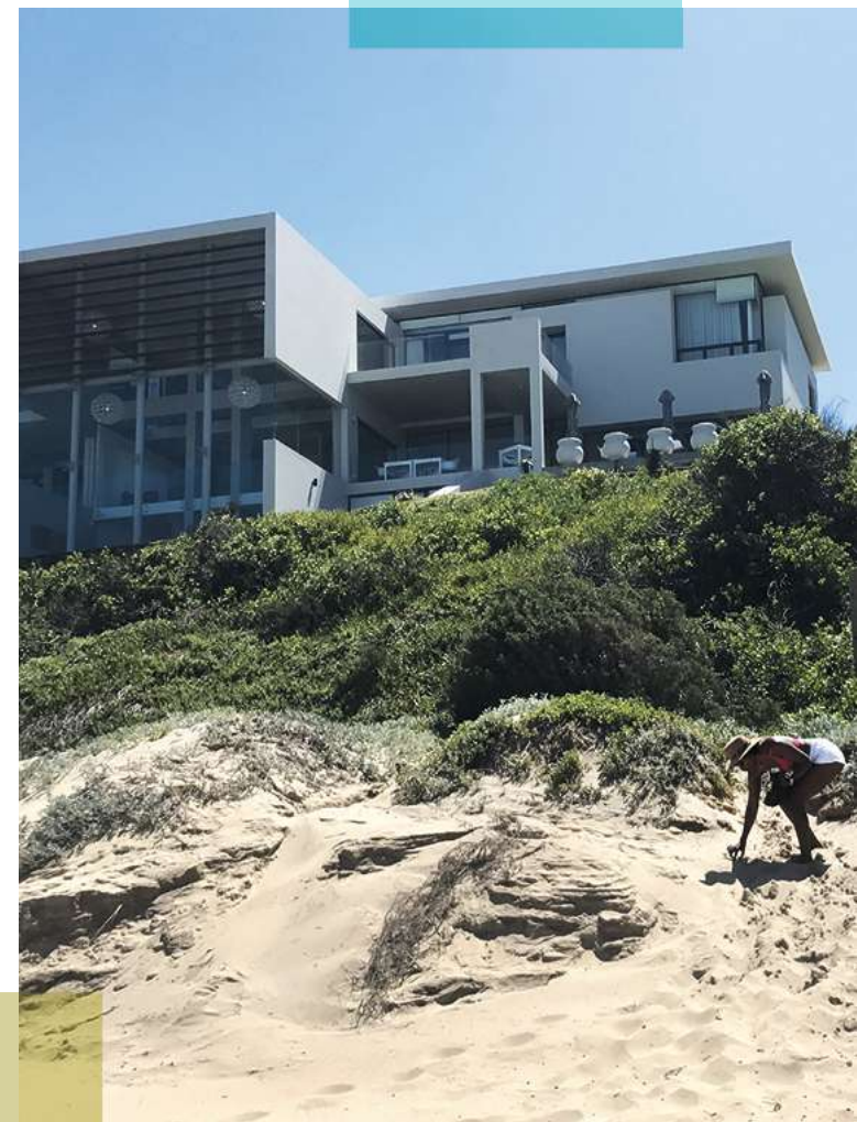
BIOROCK showed 99 percent cleaning efficiency at a holiday home in South Africa.
