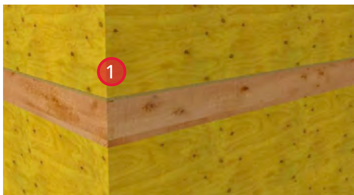
1. Typical wood frame construction at sheathing installation stage.
