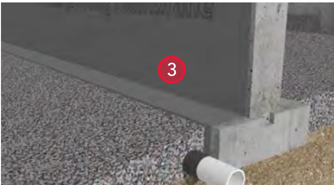
3. Install perforated pipe with filter fabric at the base of the footing and fill around with drain rock.
