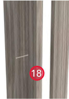
18. The window trim boards (face and returns) must be nailed together either before or during installation.
