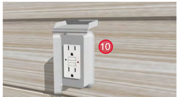
10. Install sealant around the perimeter of the electrical box (top and sides).
