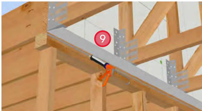
9. Apply a bead of sealant between the sheathing and sheathing membrane below the roof to increase air tightness.
