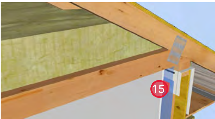
15. Install ROCKWOOL COMFORTBATT in the attic space.
