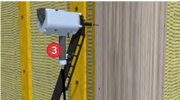
3. Install strapping as required to support the corner trim boards and cladding. Install corner trim boards.
